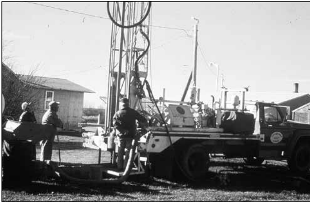
Figure 6. Test drilling to locate groundwater aquifers
