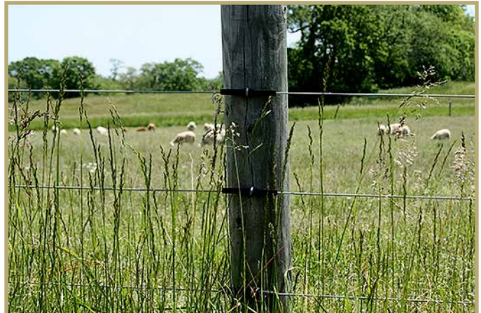
6-8. Permanent electric perimeter fence
