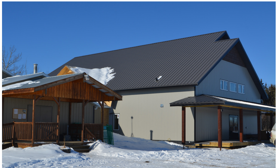
New Fourth Creek Hall under construction
